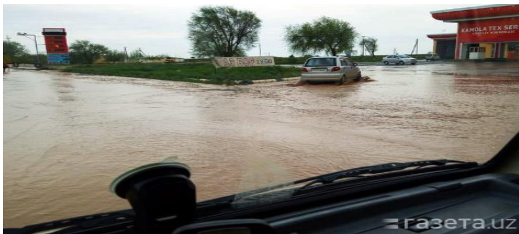
Figure 1. Consequences of flood flow affecting the infrastructure of the settlement.
