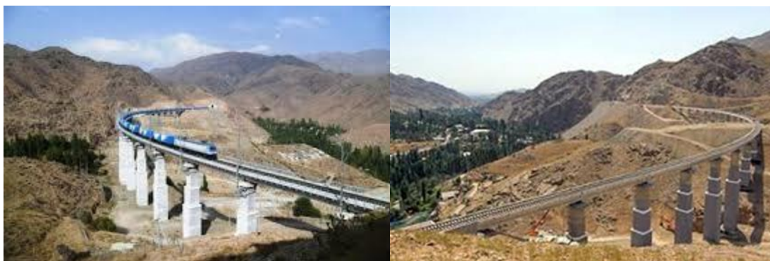
Figure 4. Steel constructed in areas with high flood risk road structures (bridges).
