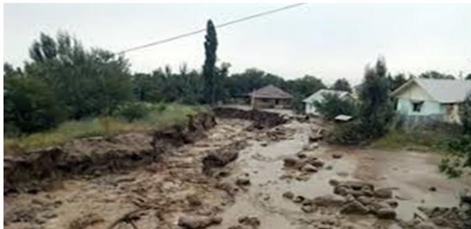
Figure 2. Post flood situation.
