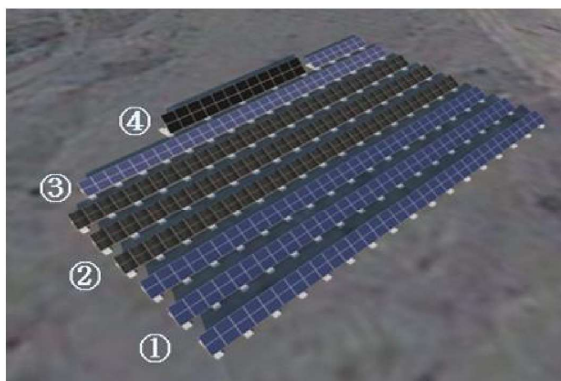
a) Rows of solar panels
