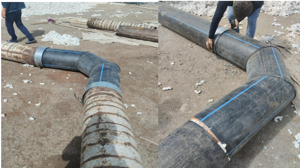
Figure 5. Introduction of the newly proposed elbow into the production process.
