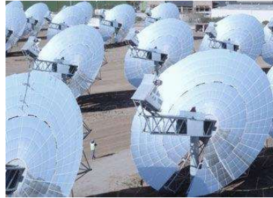
Figure 1.7. A system of generating electricity from solar energy using a Sterling engine
